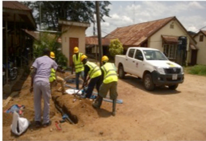
Excavation to lay the pipes
